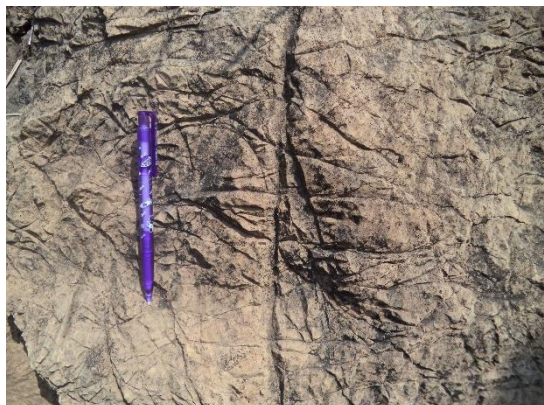
Figure 6 Highly jointed, brecciated, and criss-cross joint pattern in dolomitic limestone, Location: 96°20'7.372" E and 22° 07' 28.425" N (Facing : East)
